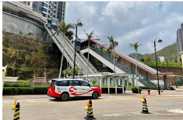
A new escalator is installed adjacent to “Toscana”, offering a direct link between DB North Plaza and the taxi stand
